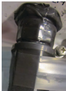
Figure 4.14. Wrapping the Connector with Rubber-splicing or Self-amalgamating Tape
