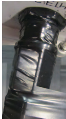
Figure 4.16. Wrapping the Connector with Electrical Tape
